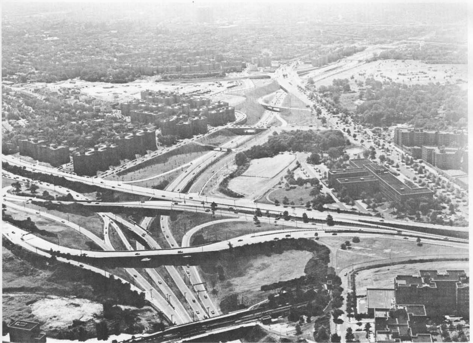
GRAND CENTRAL PARKWAY, VAN WYCK EXPRESSWAY INTERCHANGE AT KEW GARDENS
