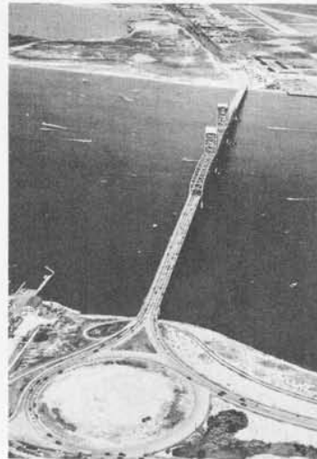
MARINE PARKWAY BRIDGE 3
