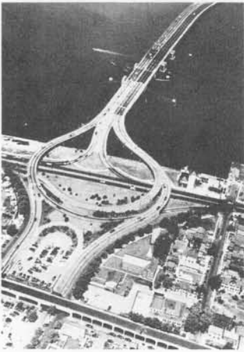
CROSS BAY PARKWAY BRIDGE 5
