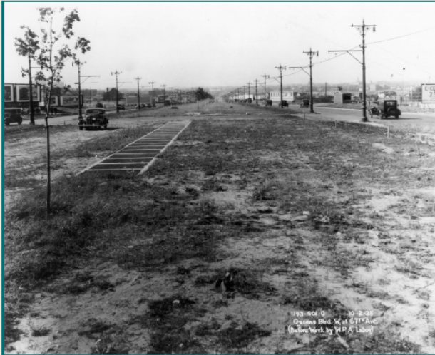
Caption: QUEENS BOULEVARD WEST AT 67TH AVENUE BEFORE WORK DONE BY W.P.A. LABOR, 1935.
