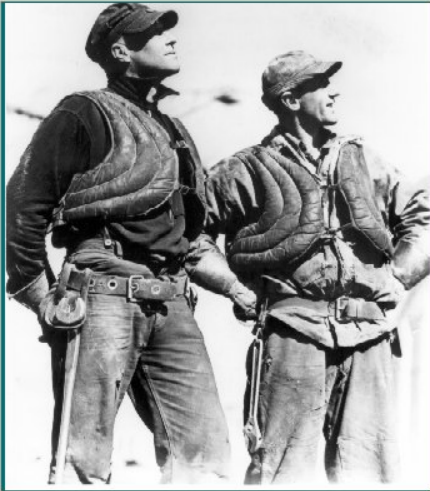
Caption: PUBLIC WORKS ADMINISTRATION RIGGERS WEARING LIFE VESTS WORKING ON THE TRIBOROUGH BRIDGE, ASTORIA, QUEENS, NEW YORK. BETWEEN 1934 AND 1936.
