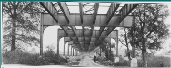
ELEVATED CONSTRUCTION ON ROOSEVELT AVE. ROUTE THROUGH ELMHURST AND CORONA. PHOTO TAKEN NOVEMBER 8, 1914.
